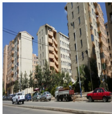
Figure 5: Fird Bet Site, Lideta Sub-City, New High Rise Condominium
