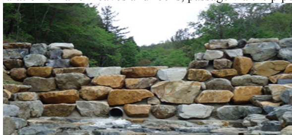
Figure 2. A check dam with structural improvement to enhance drainage
