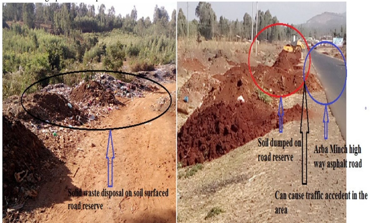
Figure 4: Soil dumped on road reserve (Source: Field survey, 2017)
