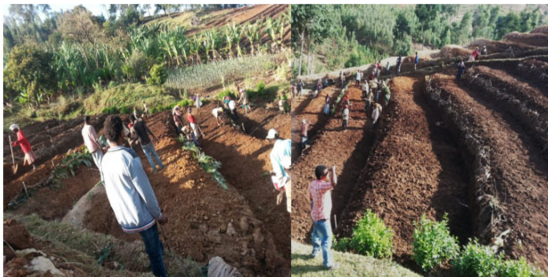
Figure2: Public campaign constructing soil and water conservation structures in Damot Waja Source: field observation photo (2016)
