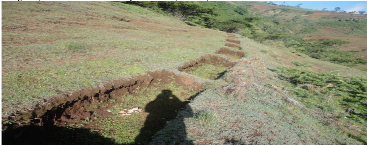
Plate 4.5: Trenches constructed on degraded land in AroWogara kebele
