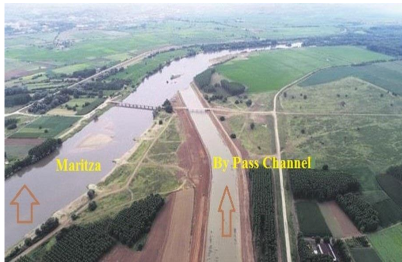
Figure 1b. Bypass Channel and Meric River.
