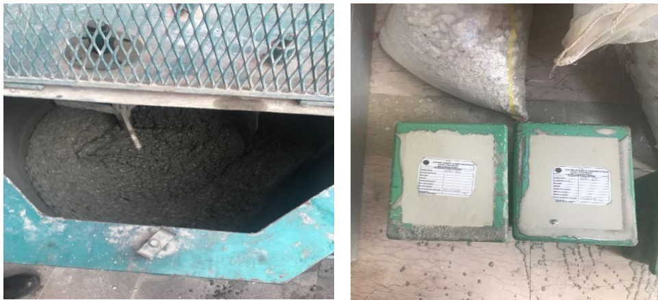
Figure 2 Mixing and placing lightweight concrete materials
