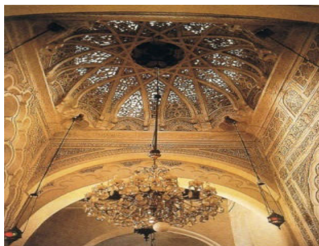
Figure (1): The Dome of the Great Mosque in Tlemcen, which is a group of cross arcs and interspersed with light from the decoration of the decorative light from the top to the bottom with decorative beams
