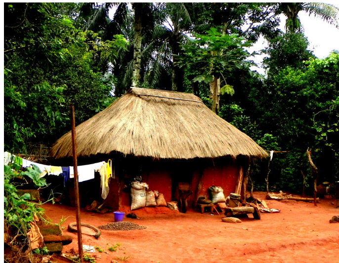
Plate 1: A Section of Thatch House
