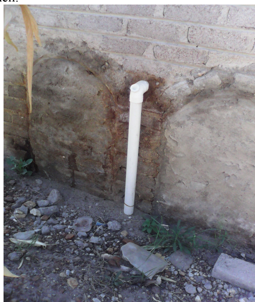
Fig 4: Outside/Backside of an Ecological Sanitation Toilet in Victoria Ranch
