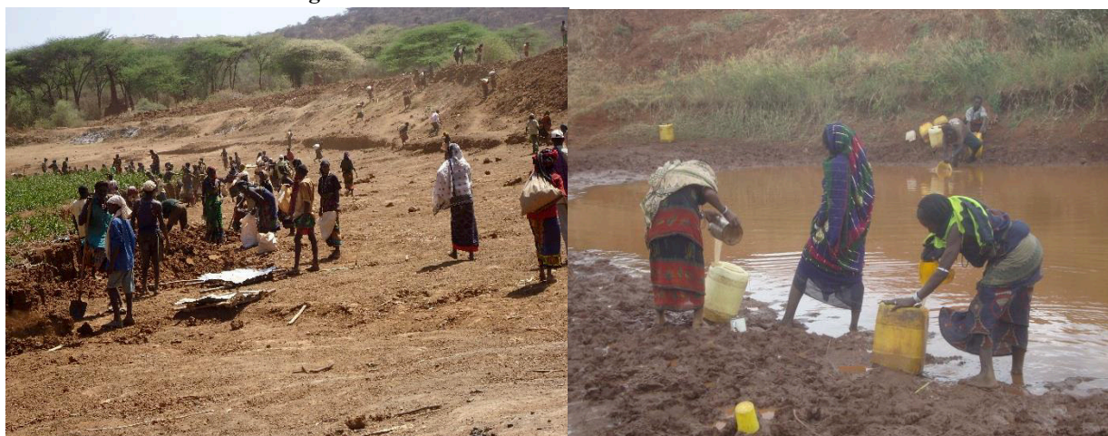
(a) Digging of shallow pond (dry season)
