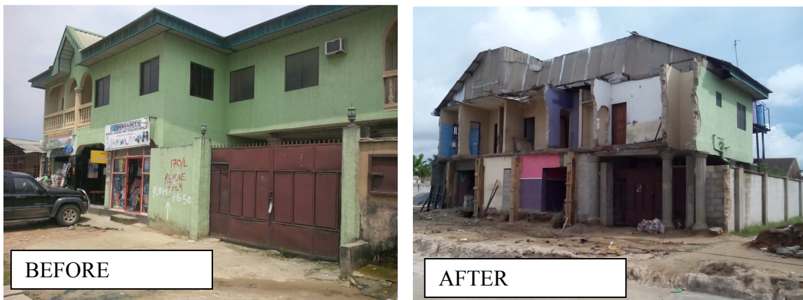
Plate 1: Picture of partially demolished residential property in the study area
