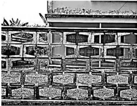
Figure 3: The use of an ornamental slab on see through top (Photo: F.M. Abejide, 2019).
