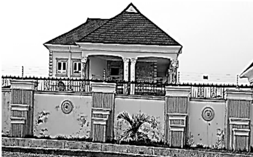
Figure 14: High fence adorned with rows of repeated triple pilasters and welded iron with tree and crown motifs (Photo: Foluso Abejide, 2019).
