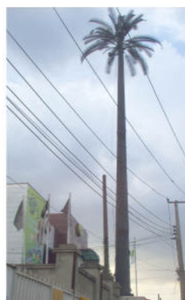
Plate 17 Globalcom mast in the form of palm tree, fibre glass, 2006, Challenge, Ibadan. Photograph: Akintonde Moses, 2008
