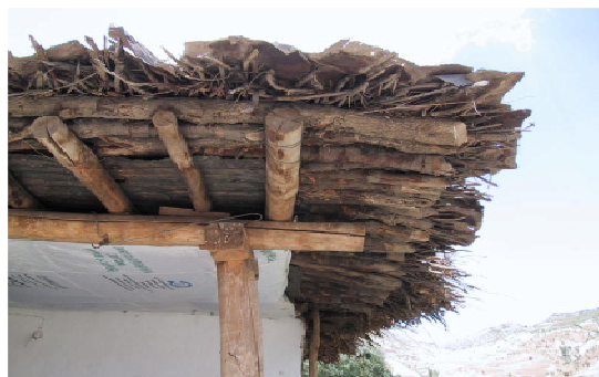
Figure 9. Roof of house in a mountainous rural area
